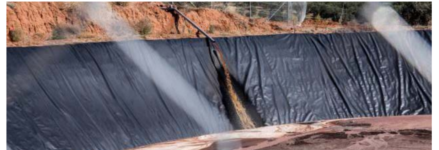
Olive Mill Industry Wastewater Treatment
