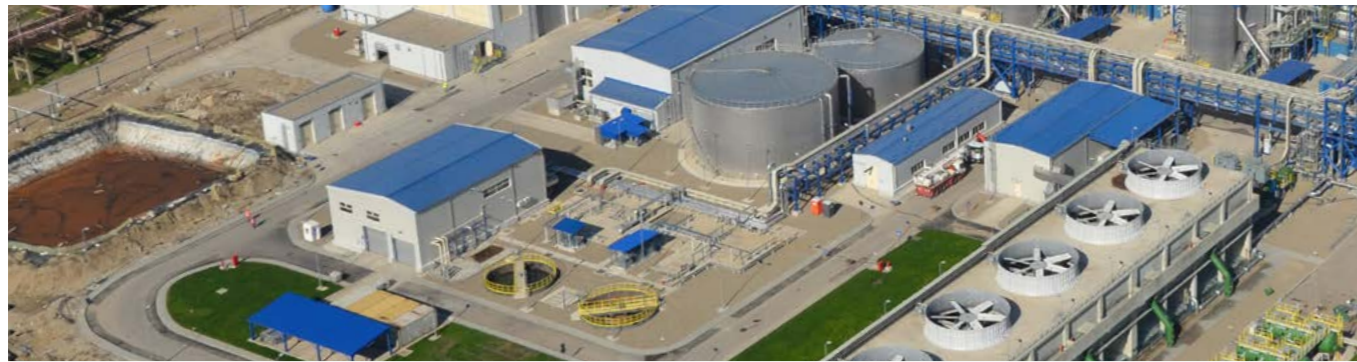
Industrial & Hazardous Waste-Water Treatment
