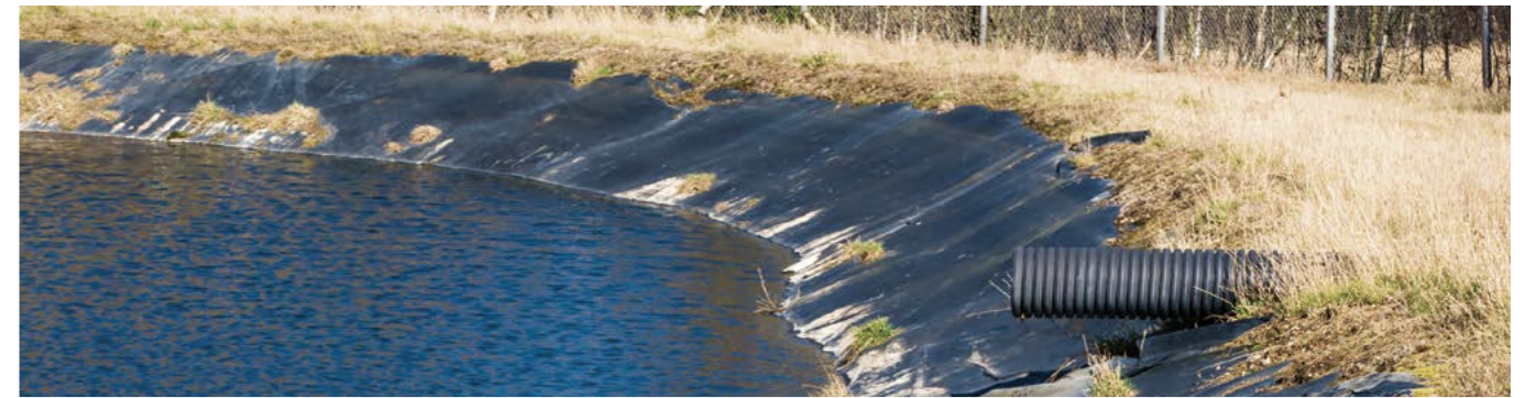
Landfill Leachate Treatment
