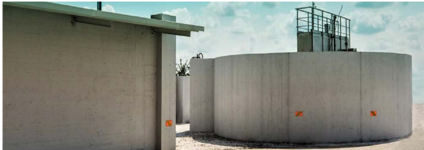
Metal Industry-Anodizing Plant Wastewater Treatment
