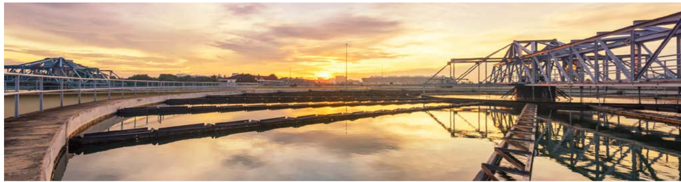
Municipal Waste-Water Treatment
